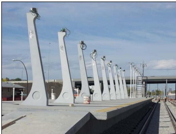
After erection, the columns were aligned, the anchor bolts connecting the columns to the cast-in-place platform cross beams were tightened, and the gaps between the column bases and the cross beams were grouted with a high strength, non-shrink grout. After erection of the columns, temporary scaffolding was erected to support the canopies and position them at their proper elevation and alignment.
