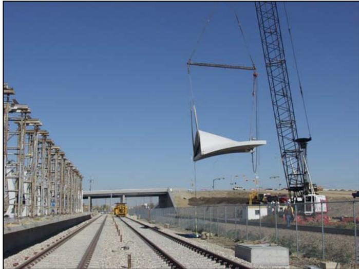
On site, the canopies were lifted onto temporary supports and adjusted to their proper alignment and elevation. Once the canopies were installed, the struts were lifted into position using the assembly frame as support for the chain hoist.
